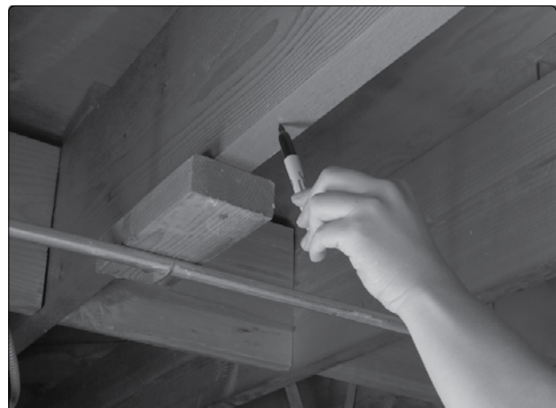
6b Mark structural ceiling for lag bolt installation
